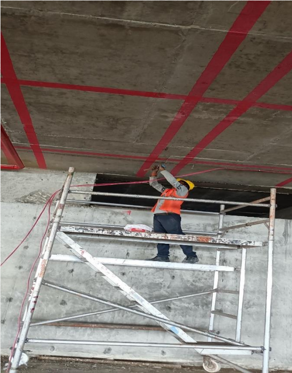
Tower -A L-27th floor Fire alarm cableing work in Progress
