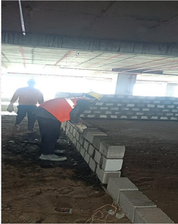
TOWER-A L-22nd floor Brick Work IN PROGRESS
