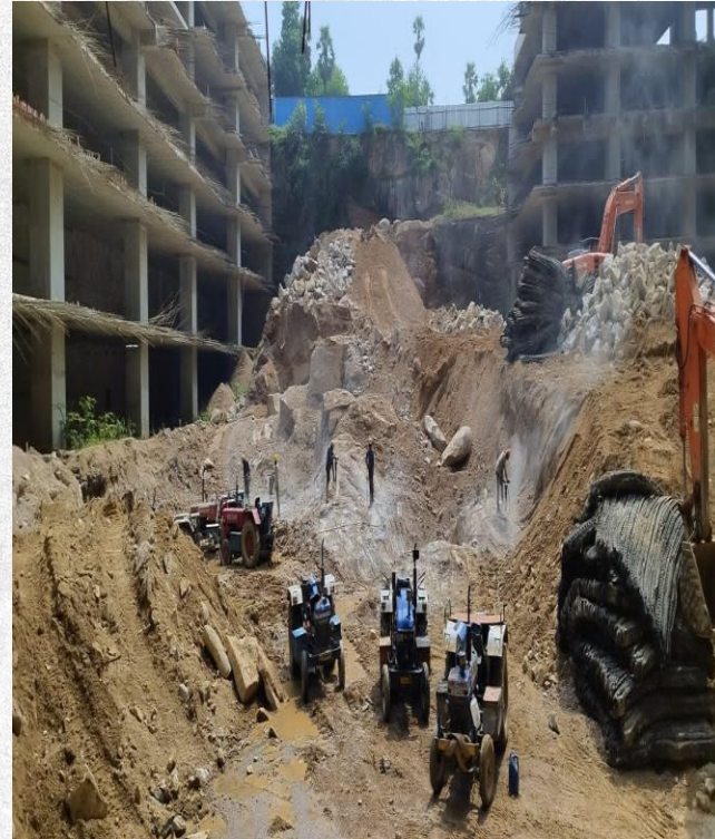
Tower B B5 Excavation work in Progress
