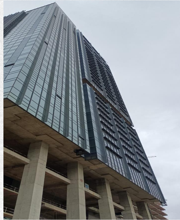
Tower A South View
