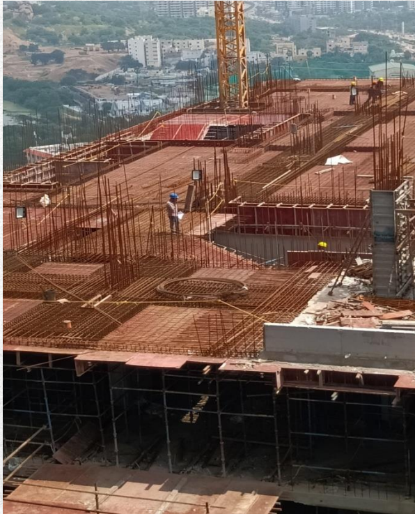
Tower C level 19th floor reinforcement works in progress
