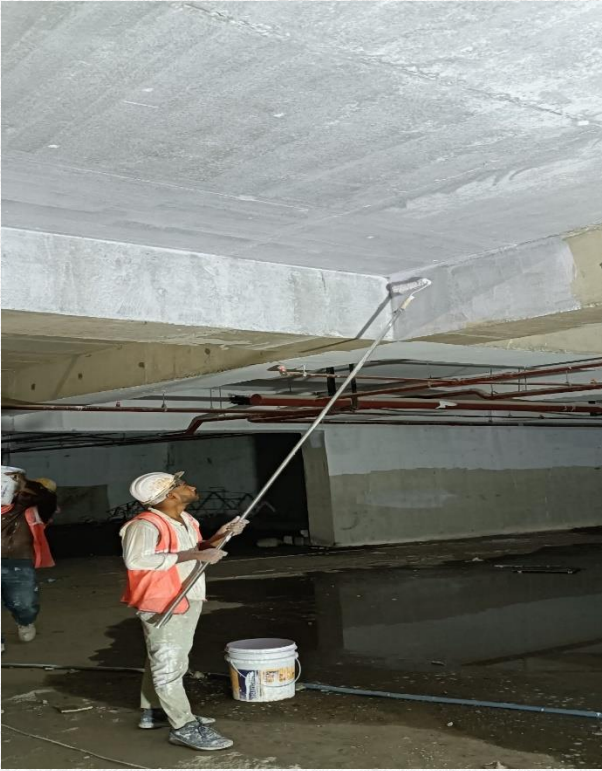
Basements-02 ceiling painting works in progress
