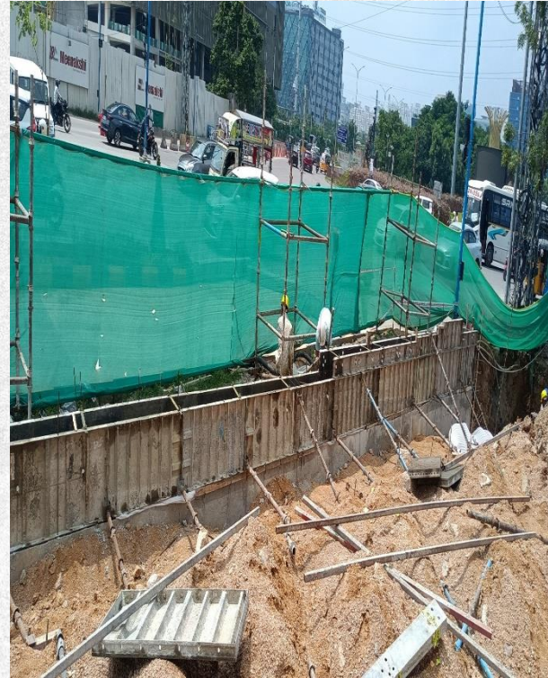
Ground floor:External Trench work in progress
