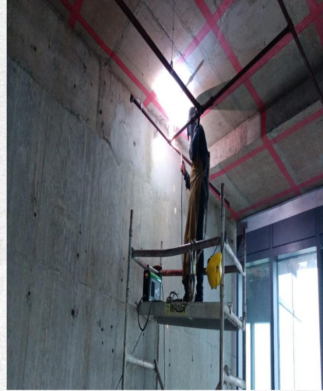
Tower A level 18th floor FPS welding work in progress
