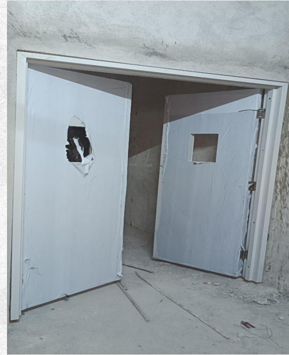
Tower-A L-22 Fire door fixing works in progress
