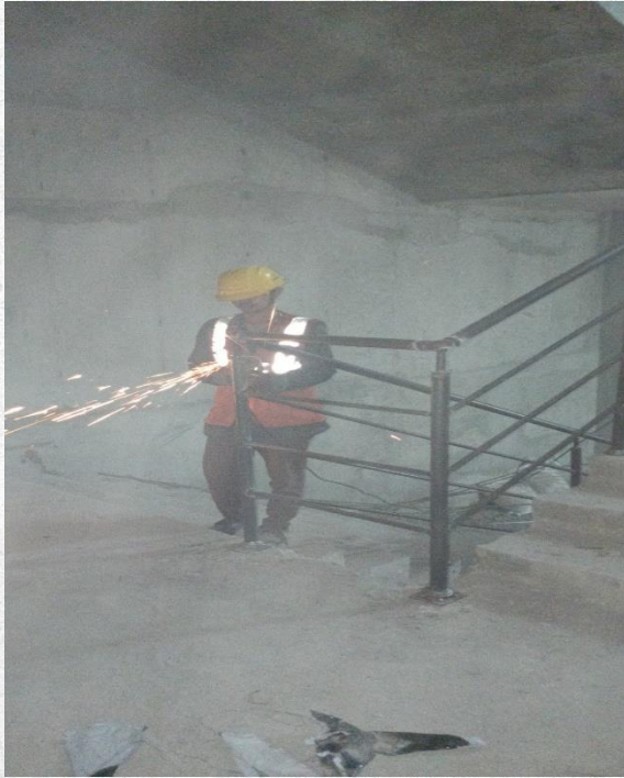
Tower -A L-01 St-03 hand railing welding works in progress
