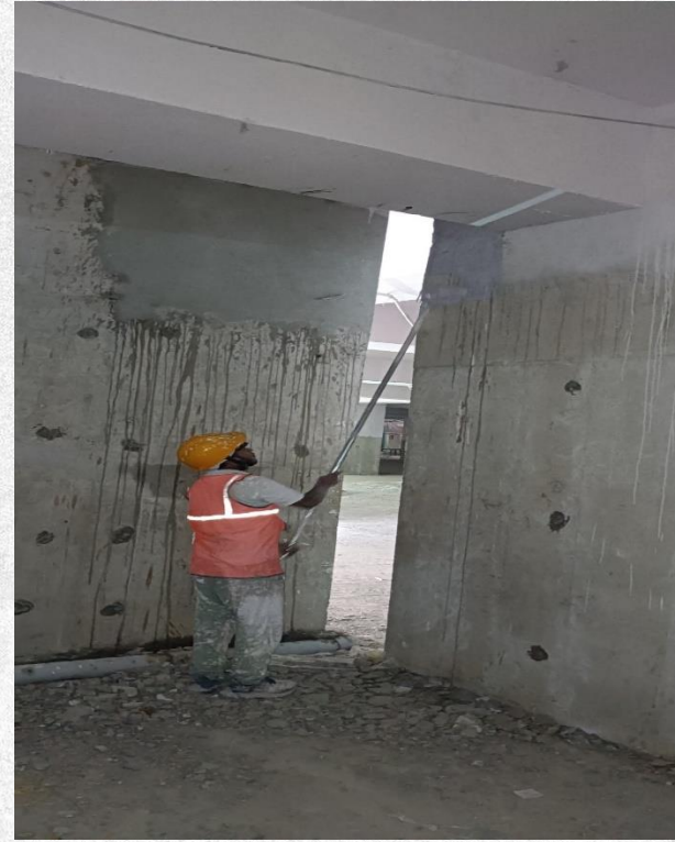
Basements-01M painting works in progress near KLC store area.
