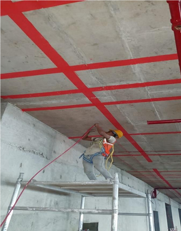
Tower -A L-24th floor Firealarm cableing work in Progress
