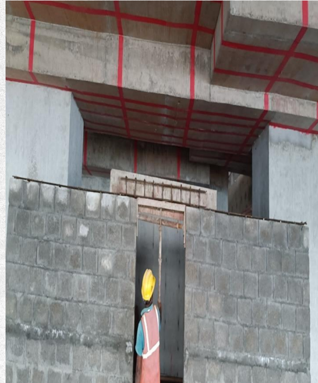
Tower C L-10 AHU room lintel work in progress
