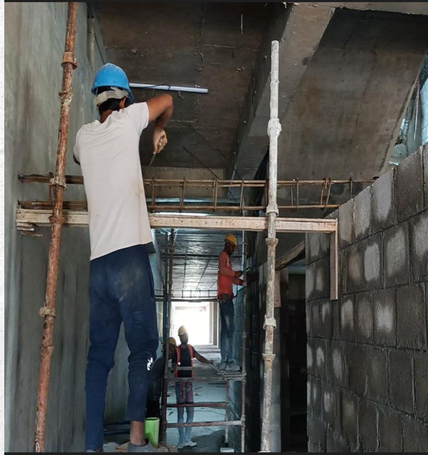
Tower -A L-2 Brick work near Staircase -01 in Progress
