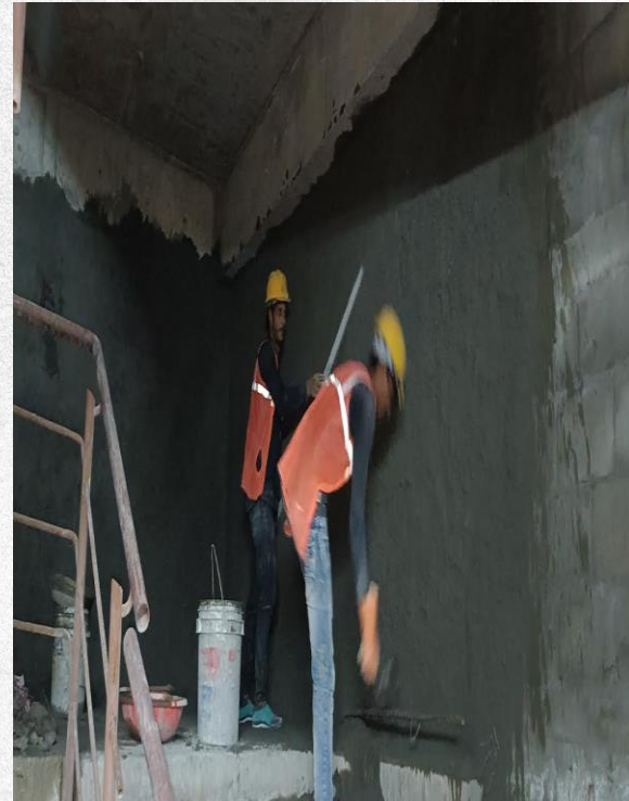
Tower A stair case plastering work in progress
