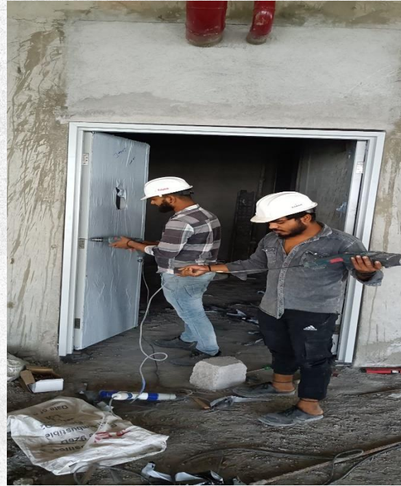
Tower-A L-28 Fire door fixing works in progress
