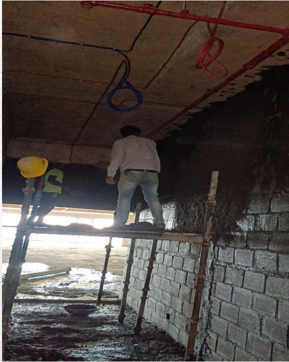
Tower -A L17 plastering work in progress
