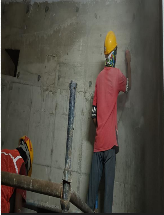
Basment-02 wall buffering works in progress
