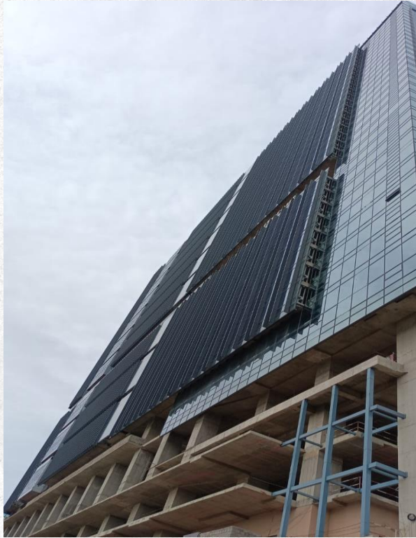
Tower A North View
