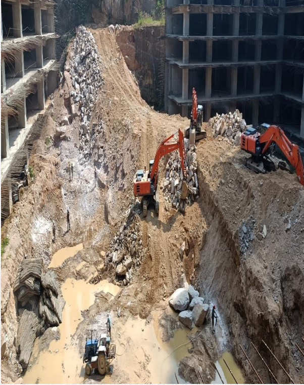
Tower B B5 Excavation work in Progress
