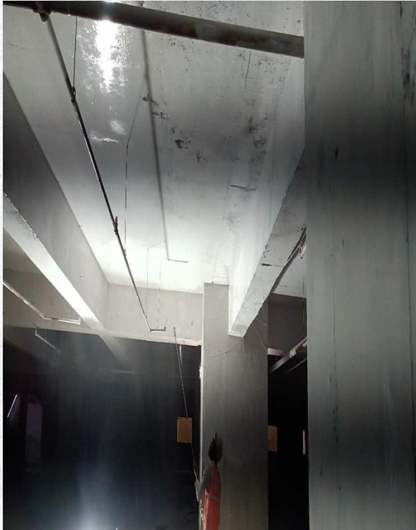
Basements-02 ceiling painting works in progress
