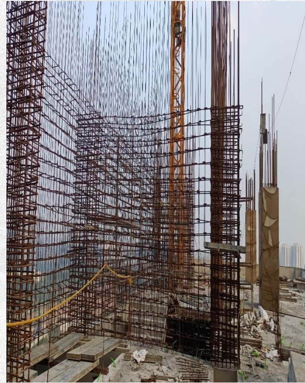
TOWER-C L-20 steel reinforcement work in progress.
