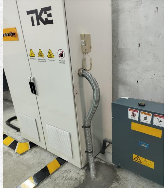
Tower-A FS-03 L-38 floor painting works
