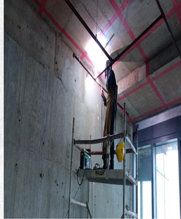
Tower-C L-20 shuttering works in progress.
