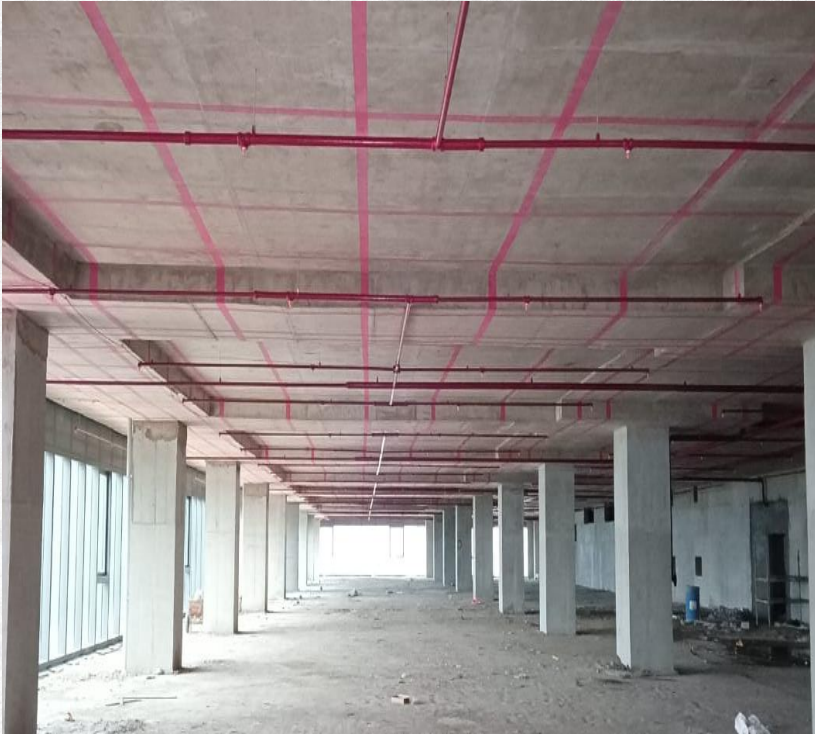
Fire Piping Installation In Level -28 and above(TOWER-A1)
