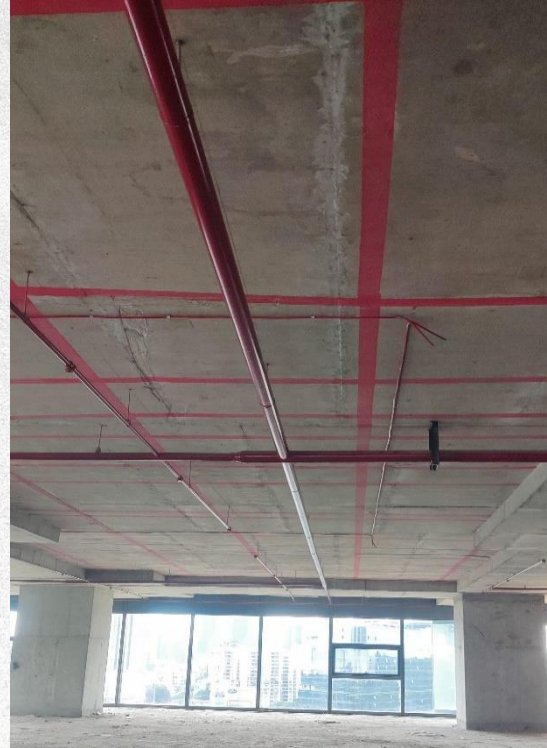
Fire Alarm cabling works at various levels in TOWER-A1
