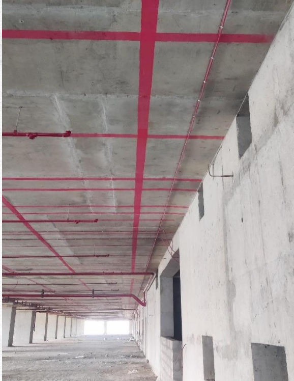
Fire Alarm cabling works at various levels in TOWER-A1
