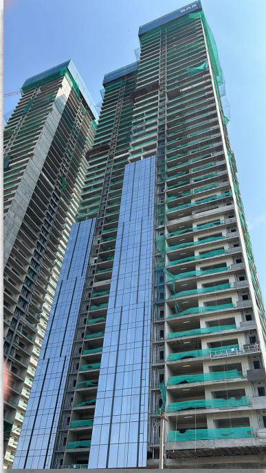
Tower 1 - Completed till L-24 Tower 2 - Completed till L-23
