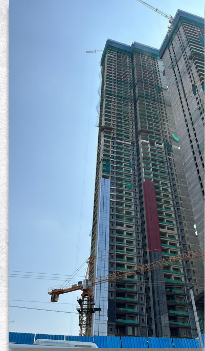
Tower 4 - Completed till L-25 Tower 5 - Completed till L-25
